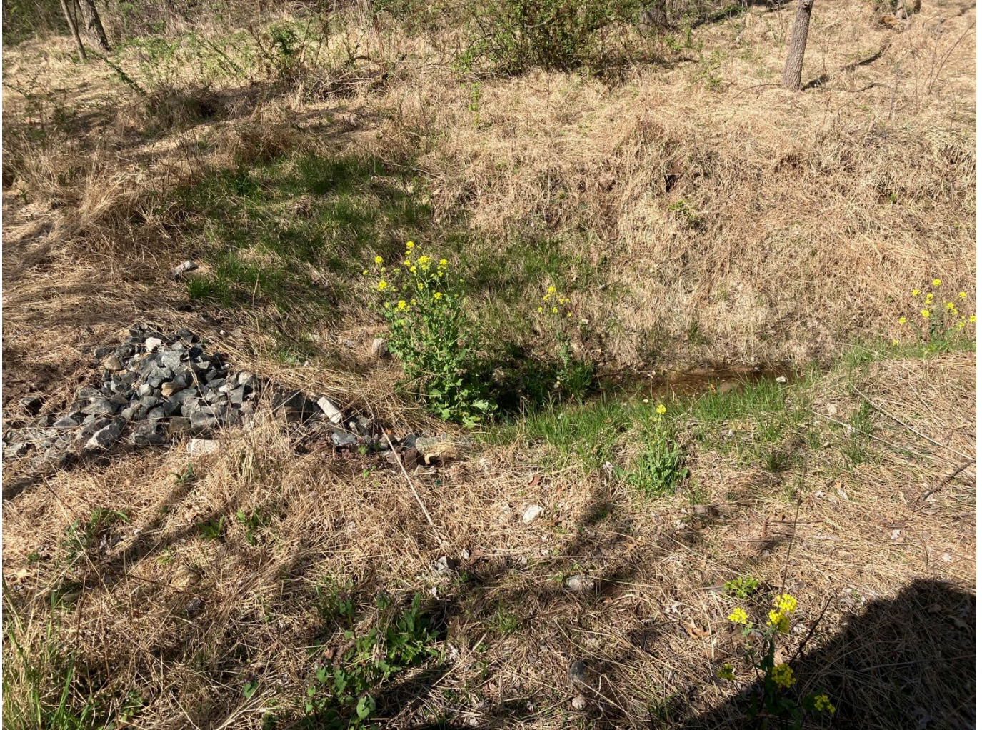
Restored stream crossing, removal of building debris and stabilization of erosion.
